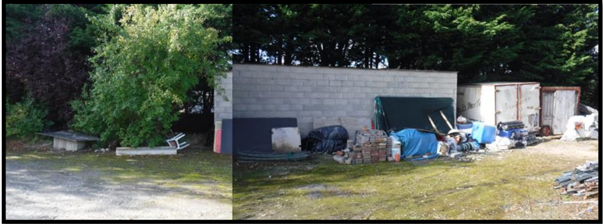
Figure 7: Existing unauthorised building on site
