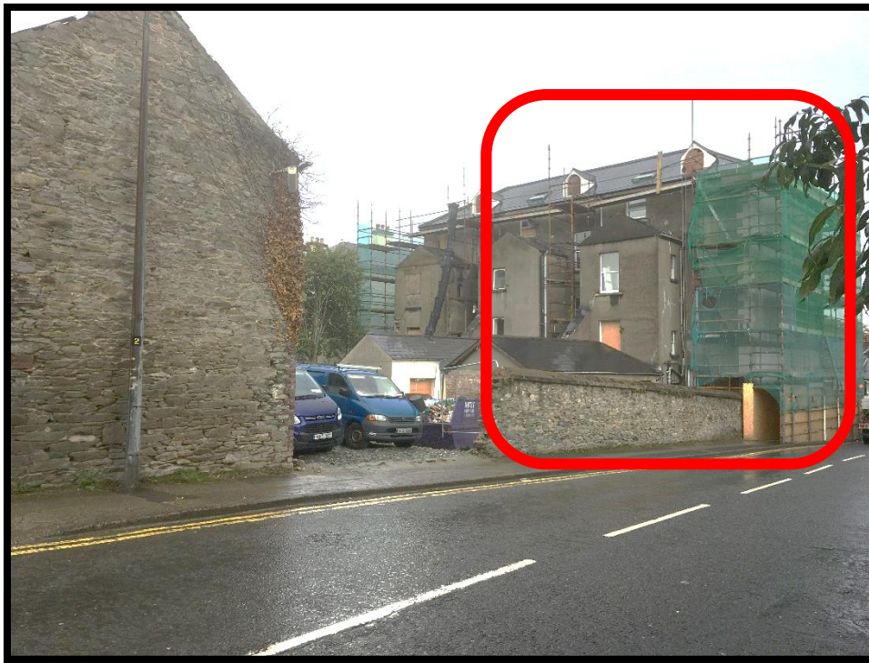
Rear elevation from Eden Terrace
