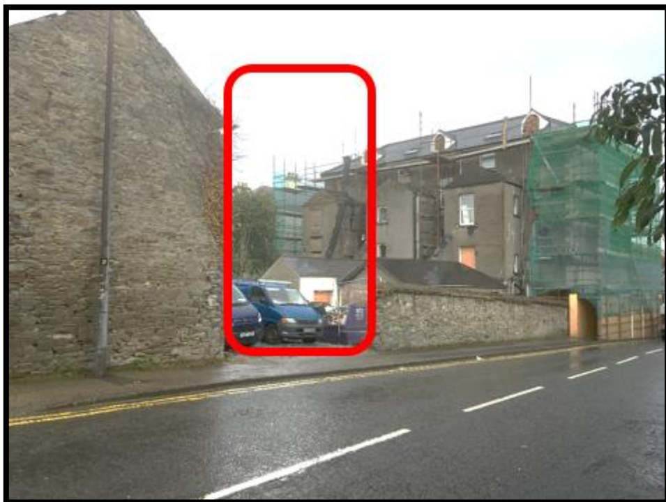
Rear elevation from Eden Terrace
