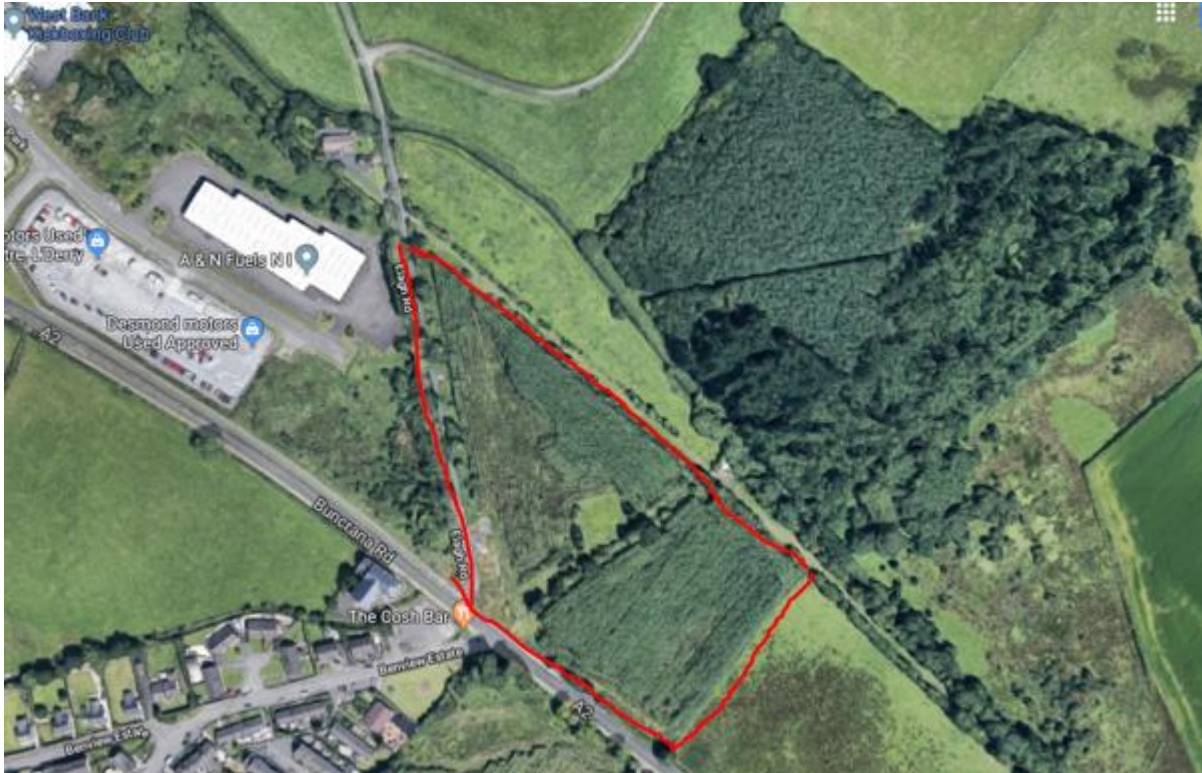
Aerial Photograph of Site
